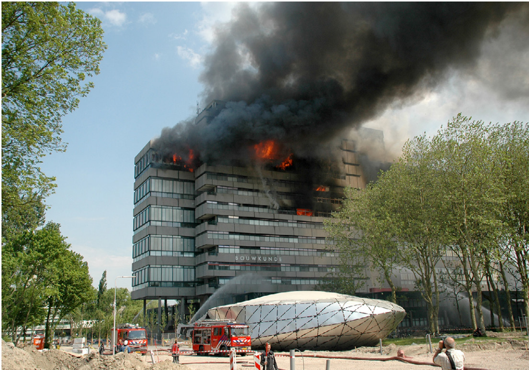
Figure 5: Fire in a high-rise building (University of Technology Delft, The Netherlands)
