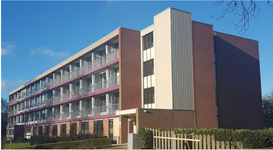
Figure 1.1: Residential building in Oudewater in which the experiments took place
