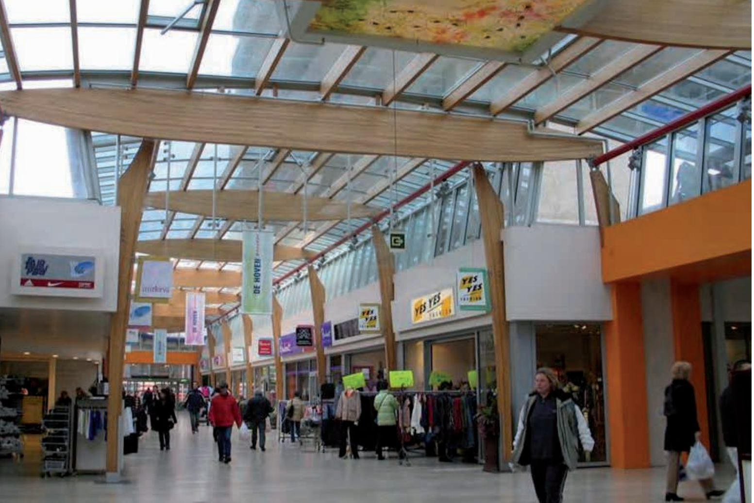
Risks of large non-compartmented surfaces
