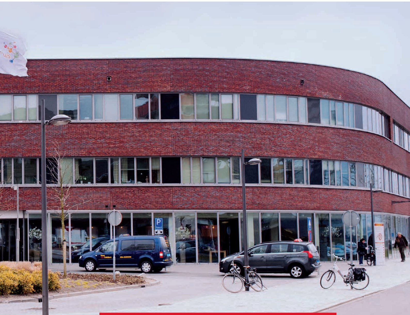
Building group 3: people who are not able to leave without assistance, sleeping / e.g. a hospital
