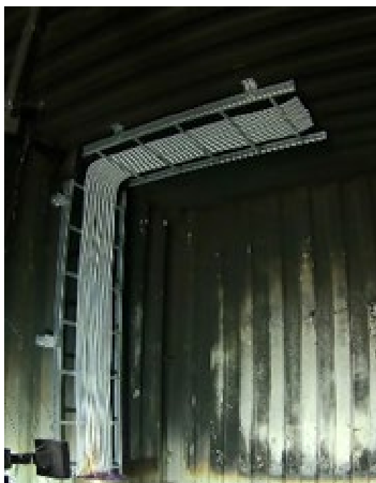
Figure 2.20 Fire size high performance cables after 3 minutes
