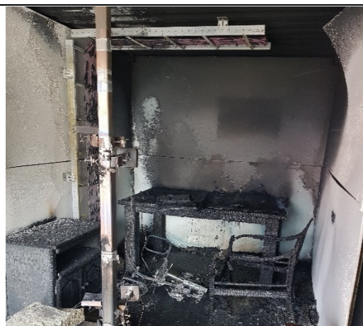
Figure 3.7 Office after the test
