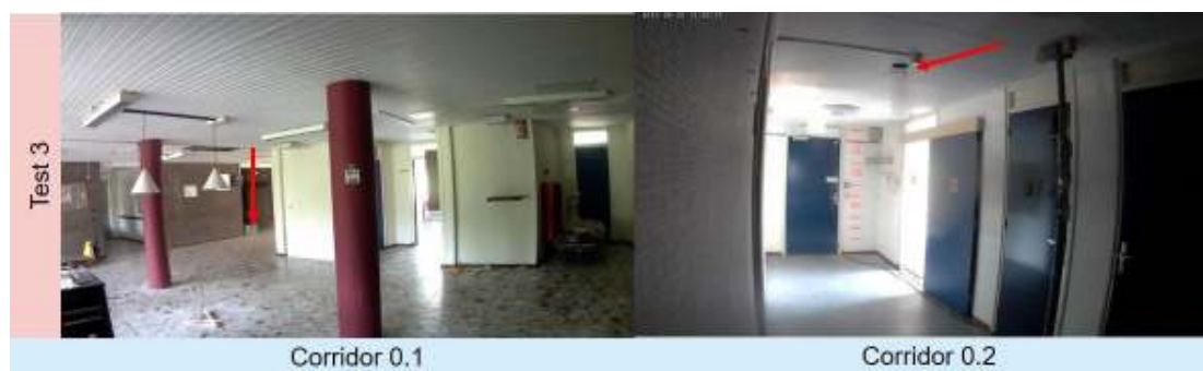
Figure 3.22 Smoke propagation to the ground floor during test 3 of variant 0
