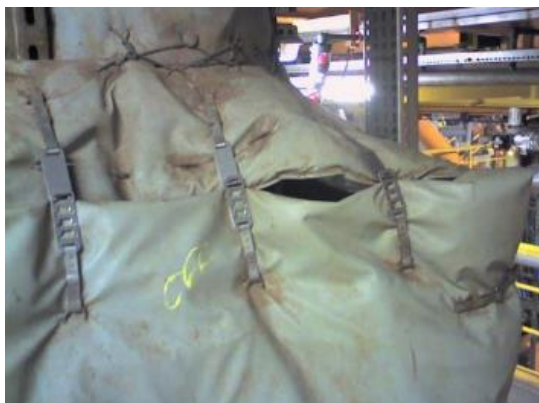
Figuur 24 - Open scharnier in jacket-type dry-fit systeem
